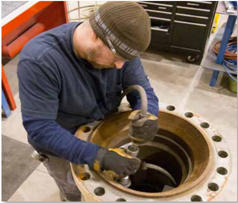
Valve cleaning & inspection
