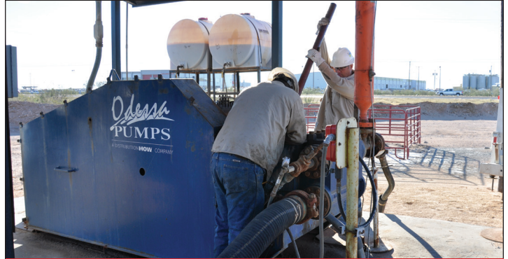
PLUNGER PUMP REPAIRS
